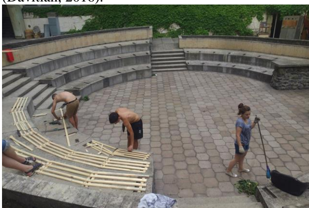
Photo 1. Initial stage of “Colosseum” revitalisation
